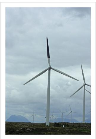
FIGURE 2 A wind turbine in the Smøla wind-power plant with one rotor blade painted black. © Roel May.
