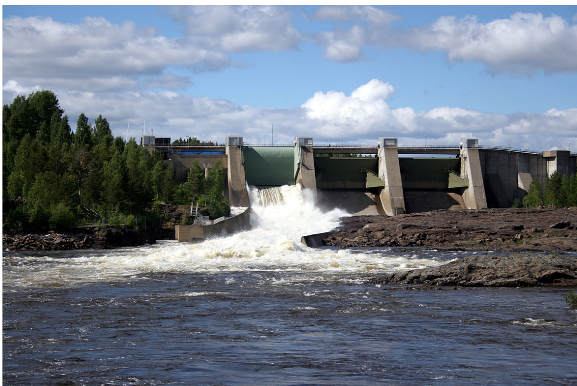
Photo: Stornorrfors dam, Umeå. Source: sv.wikipedia.org
