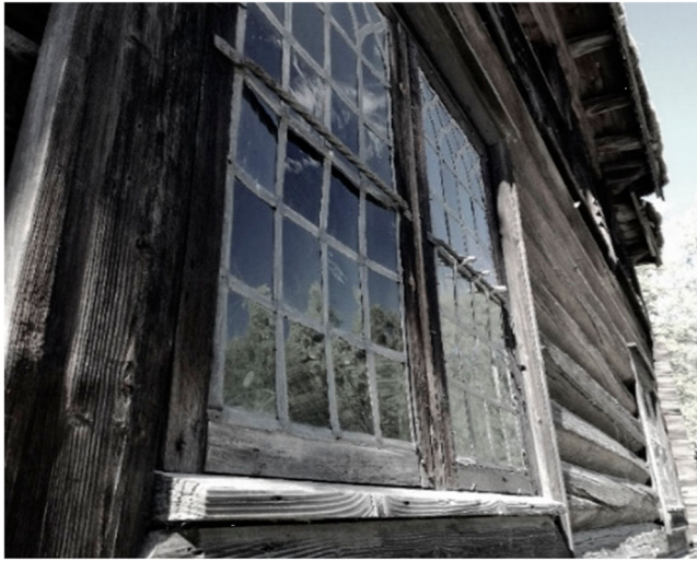
Figure 3. Photo taken by a 64-year-old man from Norway.
