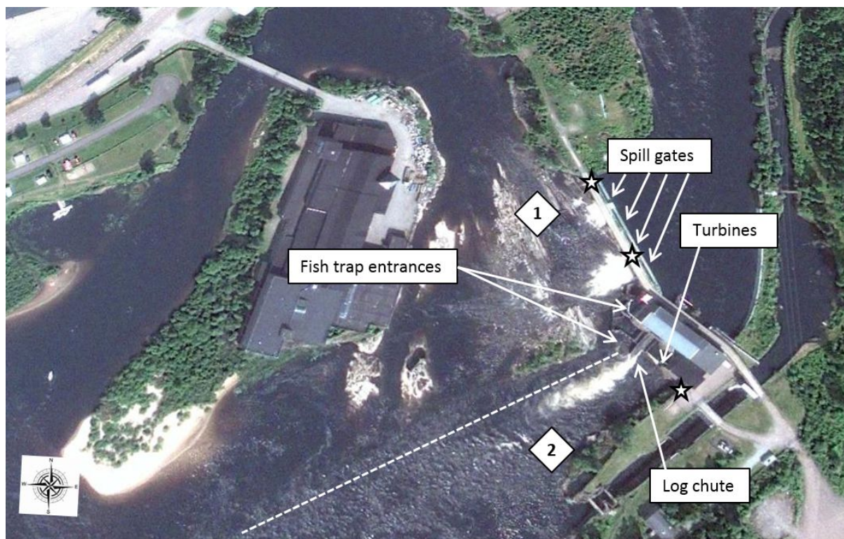
Figure 3. Aerial photo (google maps) of the power plant at Forshaga, River Klarälven, showing the location of the three turbines, four upward-opening spill gates and one downward-opening log-chute. There are two entrances to the fishway. The area depicted with “1” represents the spill area, and by “2” the turbine outflow area, with the dotted line showing the border between the two areas. The three stars show the location of the telemetry antennas.
