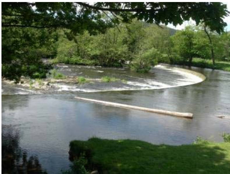
Figure 23. Horseshoe Falls. The floating log in the foreground (which functions to guide floating vegetation over the weir) marks the entrance to the Llangollen Canal, to left of shot. Beavers dispersing downstream would find it easier to enter the canal than to traverse the weir unless preventive measures were applied.
