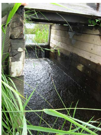
Figure 27. The stream exit from the pond by the main hide, running below the boardwalk. Currently impassable to beavers, if the step over which the water flows were converted to a ramp it would connect to good quality habitat on the downstream ditch and river Teifi.
