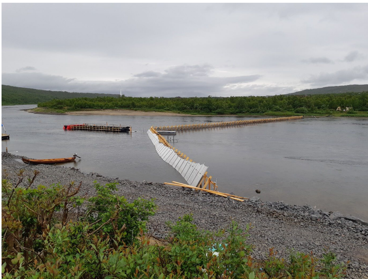
Figure 16. The fence-trap system in the eastern channel of the Tana at Seidaholmen (Tana bru). A second fence (flexible fence) was utilized in the western channel. Photo: Panu Orell.
