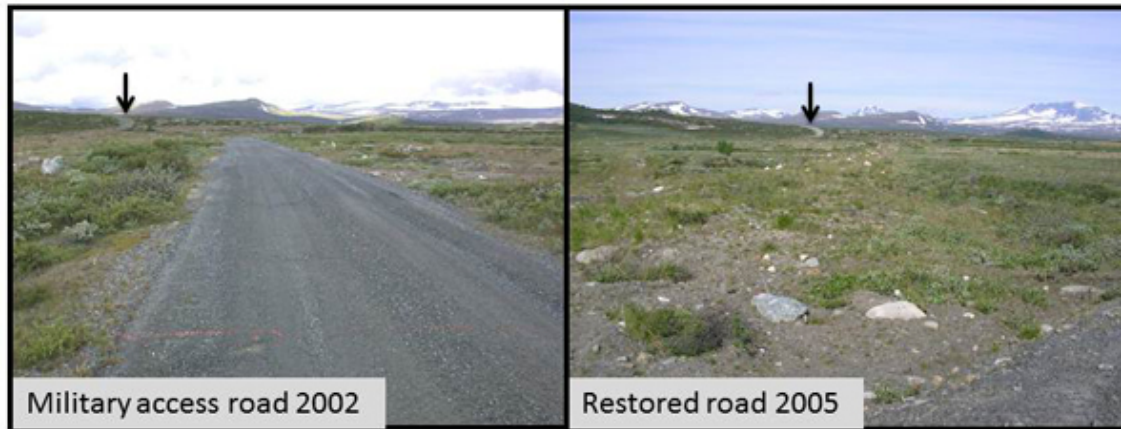
Fig. 4. Restoration of military access road (width of road is 5 m) by removing added gravel and stone, stirring the original topsoil, and transplanting turfs from the road margins. Left: the road before restoration (2002). Right: the road three years after restoration (2005). The arrow indicates a fixed point for comparison between the pictures.
