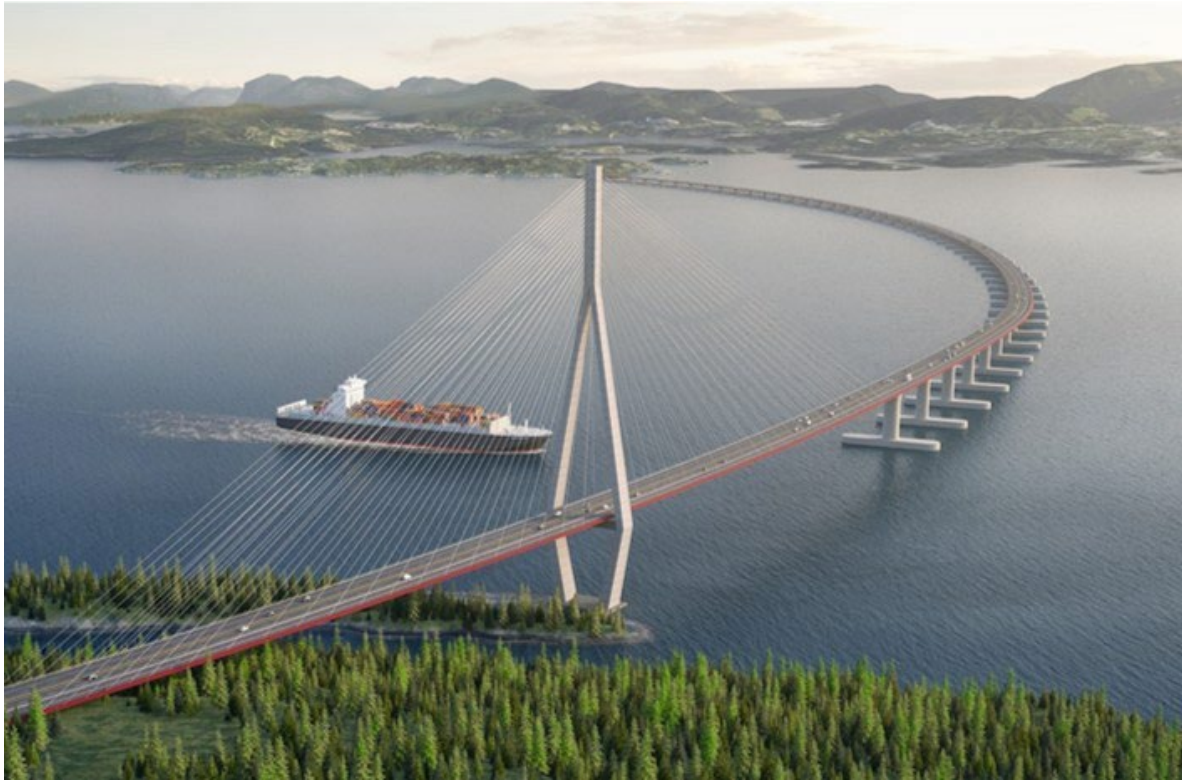
Figure 1. Floating bridge crossing Bjørnafjorden (from Statens Vegvesen).
