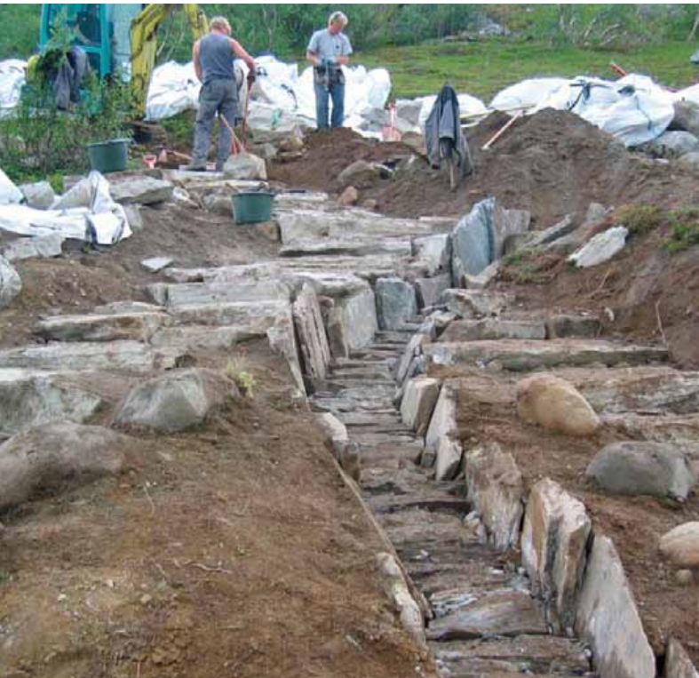
Figur 4. Vegetasjonen ble lagt tilbake etter at stien var satt i sand. - Vegetation was replaced along the path as a part of the restoration. Foto/Photo: R. Solem.
