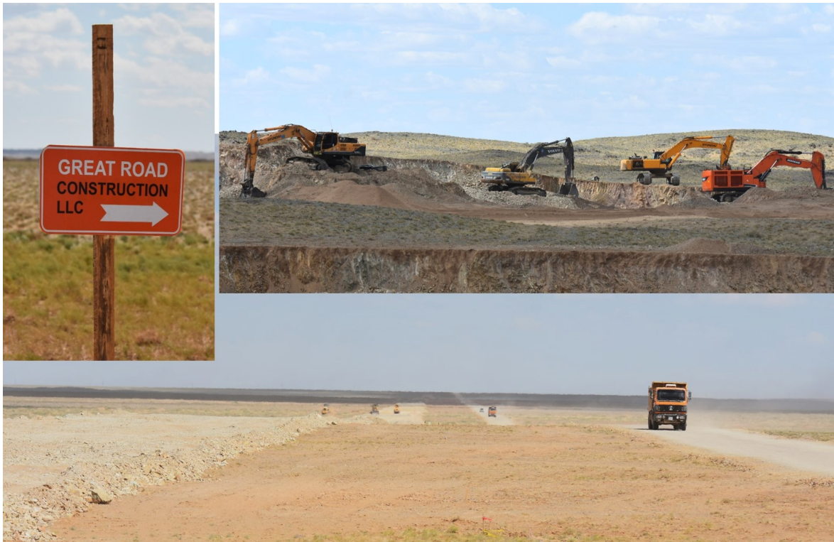
Figure 18: Railway under construction between Zuunbayan and Tsogttsetsii, August 2019. Photo: B. Buuveivbaatar
