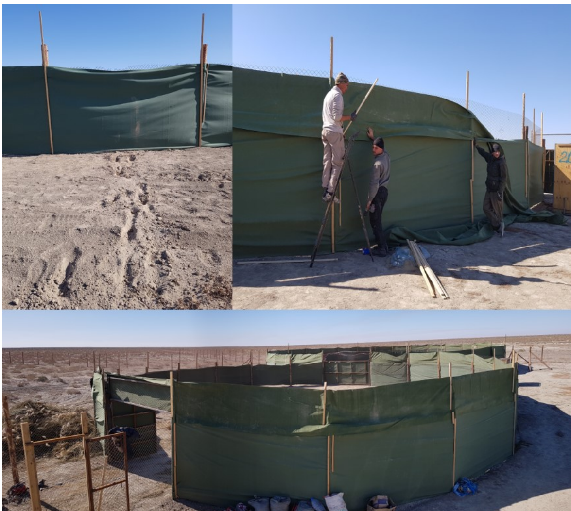
Fig. 27: Top left: Tracks of a kulan that jumped out of the 2m corral. Top right and bottom: Corral elevated to 2.7m. All kulan had to be released to allow for the 2 days necessary to implement the changes which among other work involved welding and drilling. Photos: P. Kaczensky
