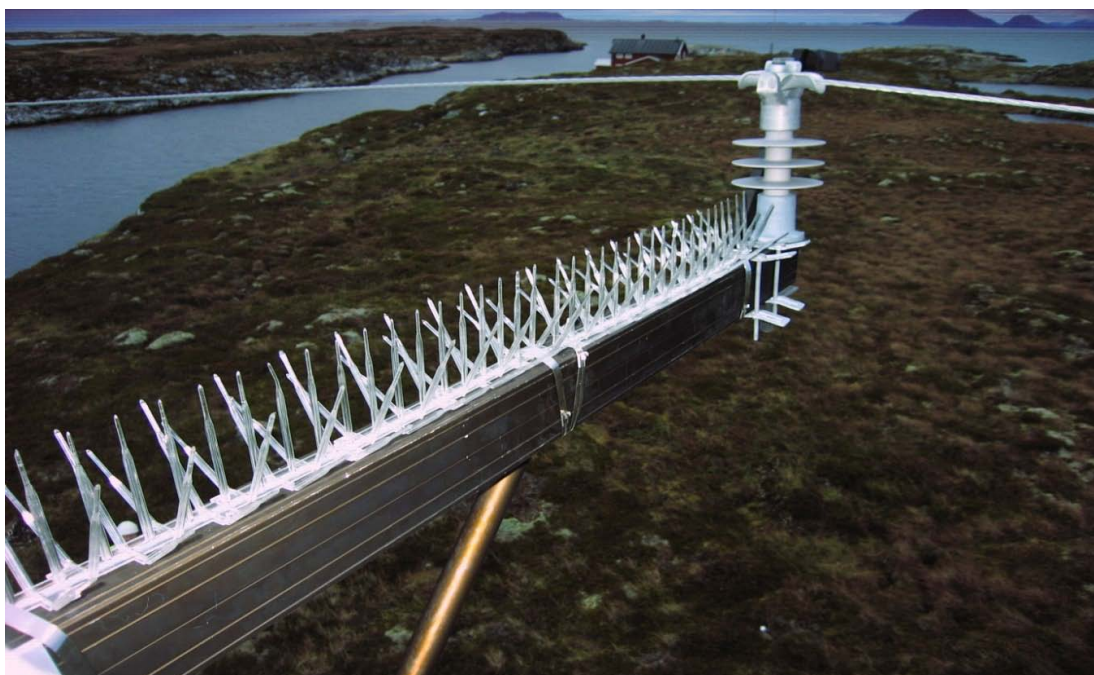
Figure 29. Anti-perch device to discourage birds perching on the crossarm. Photo Rødøy-Lurøy Kraftverk AS.
