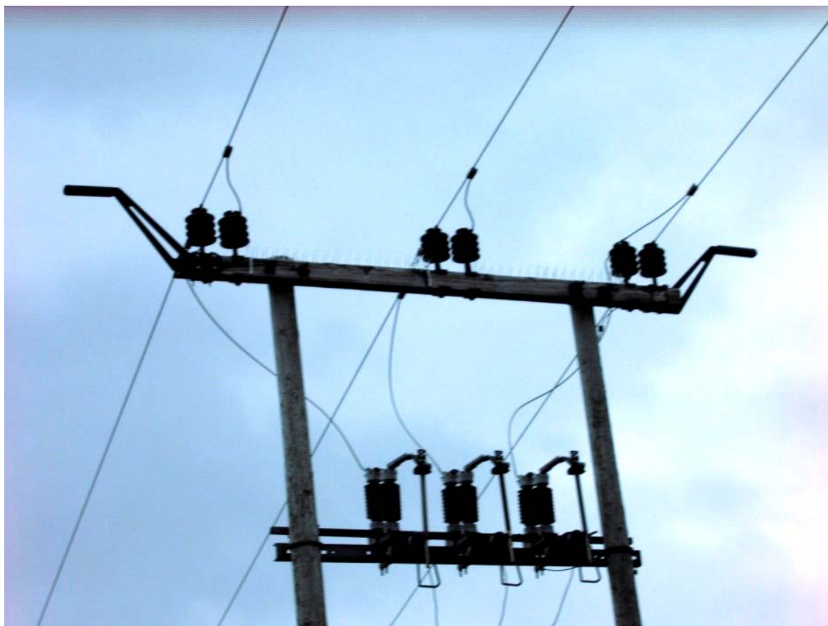
Figure 28. Deployed anti-perch device to discourage perching on top of the crossarm, and elevated perch on each side. Photo: Rødøy-Lurøy Kraftverk AS.
