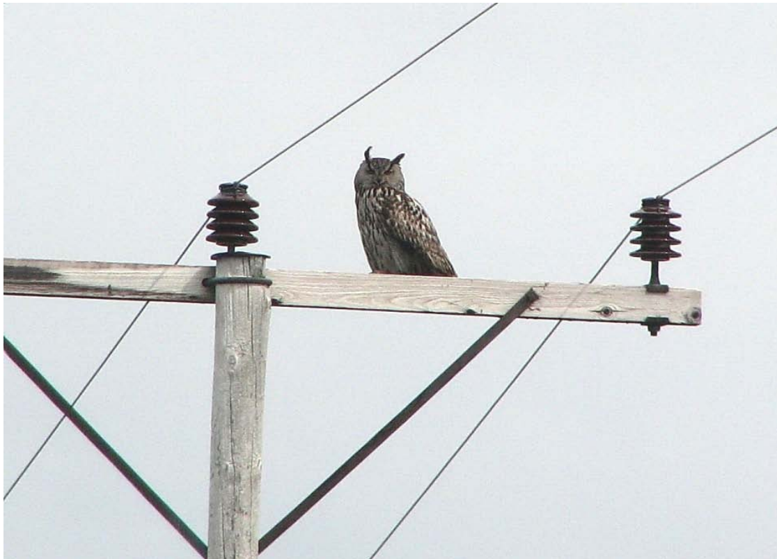
Figure 24. Eagle owls can use poles for perching during hunting. This pole has top-mounted insulators. The most dangerous poles have a grounded copper wire on the upper side of the crossarm. When sitting on this crossarm construction the eagle owl could be electrocuted when touching only one of the conductors. Photo: Jan Ove Gjershaug.
