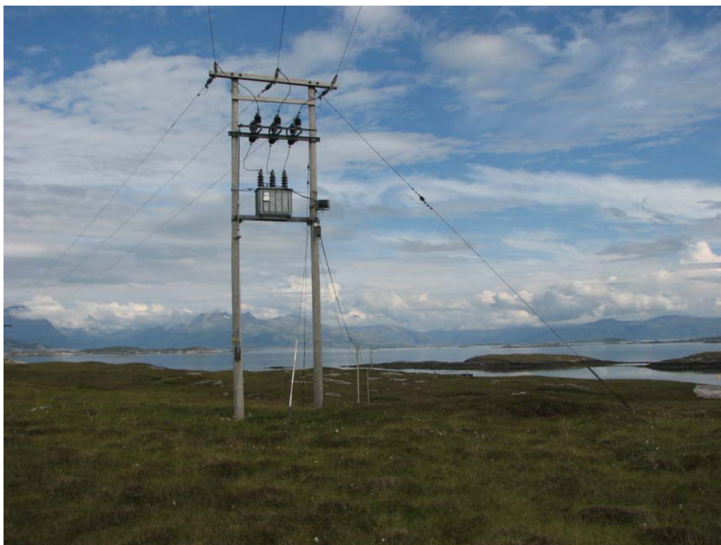
Figure 19f. Pole no 165. Pole-mounted transformer. Photo: J.O. Gjershaug.
