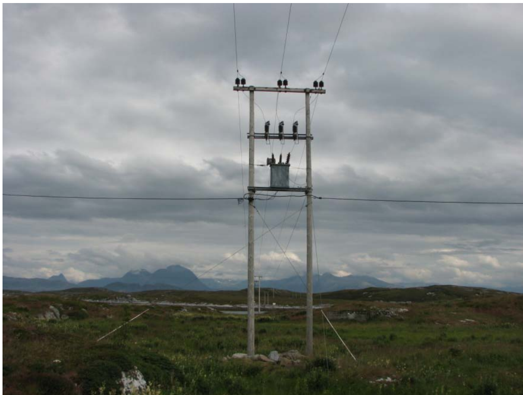
Figure 19e. Pole no 149. Pole-mounted transformer. Photo: J.O. Gjershaug.
