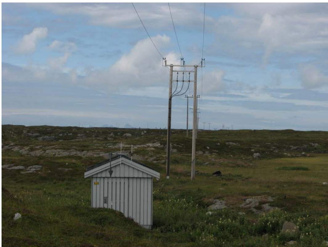
Figure 19g. Pole no 176. Cable to ground-mounted transformer. Photo: J.O. Gjershaug.
