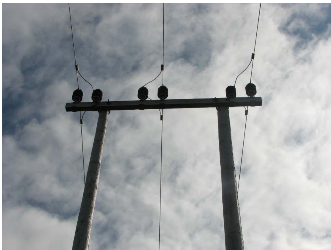
Figure 19h. Pole no 177. Double pin-isolator. Photo: J.O. Gjershaug.
