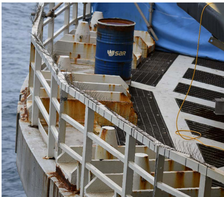
Figure 3.13. Spikes installed on Heidrun to keep gulls from resting on rails. (photo: © Signe Christensen-Dalsgaard)
