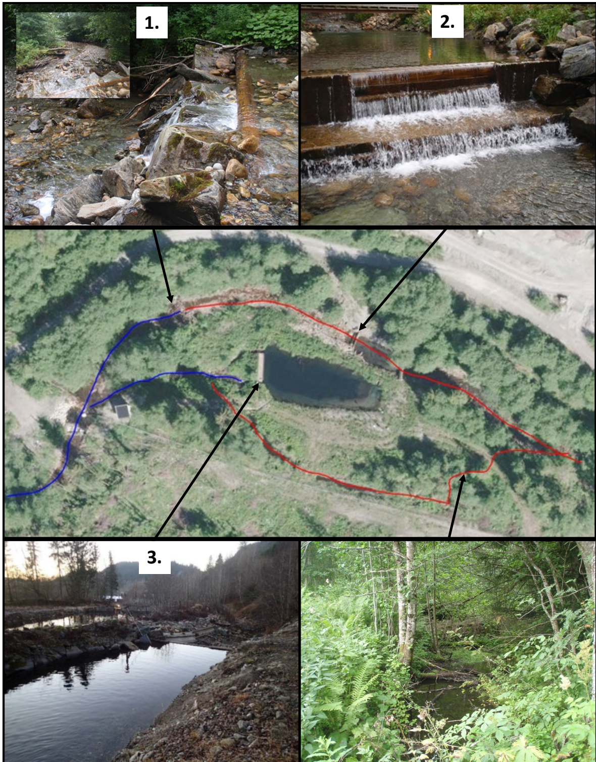
Figure 7. Location and photos of three dams in Kaldvella. The dams prevent access of anadromous fish to upstream spawning and nursing areas (inaccessible stretch shown with a red line) and cause partial drying of a side branch of Kaldvella (see photo in lower right corner). Photo: © Morten Andre Bergan. Aerial photo obtained from https://kart.finn.no .
