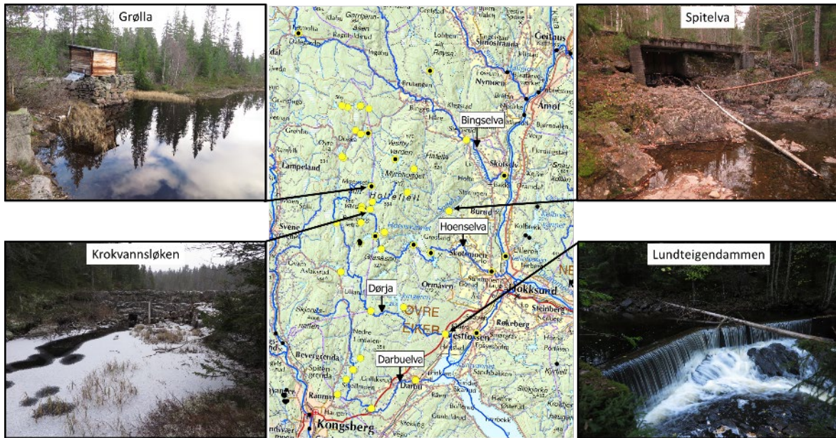
Figure 12. Potential targets for dam restorations in the study tributaries of Drammenselva in Øvre Eiker, southern Norway. Photos: © Finn Gregersen. See Appendix 4 for more detailed description.
