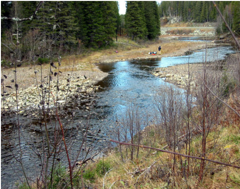
Figure 21. An example of the "river in the river" design concept in a reach with a broad stream bed where flow has been severely reduced. From the Dalåa river in the Stjørdal system, Nord-Trøndelag county, Norway. The restored reach meanders within the former river course with areas alternating between pools and riffles. Photo: Knut Alfredsen
